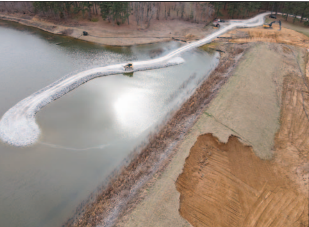
Lake George’s temporary rock dam is about halfway complete based on this aerial photo taken late last week from above the adjacent failing levee. The temporary dam will provide a safety net in case the earthen levee fails.
